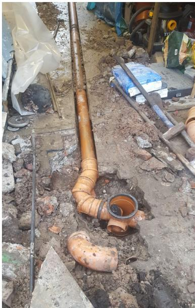
Cover new drainage pipe which leads out to connection with drain behind the garage.
