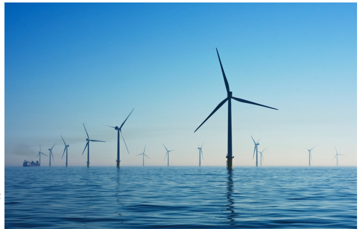
Rampion Offshore Wind Farm, UK – photo by Nicholas Doherty
