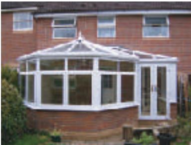
Above: the new conservatory at Binfield
