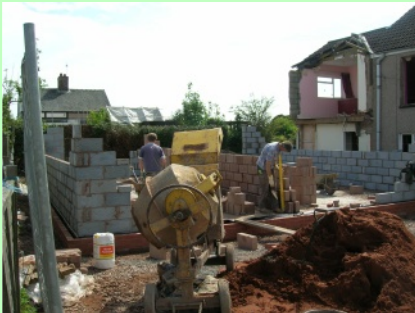
The walls go up...
