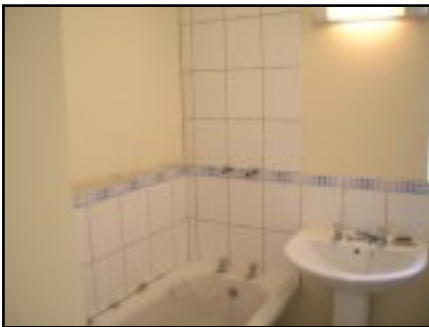
Above: new bathroom going in
