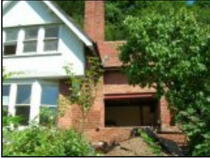
Above: Bishopswood's kitchen extension
