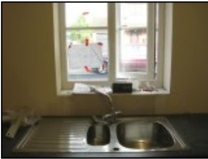
Above: new kitchen taking shape
