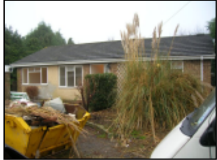
Above: progress at Lydney
