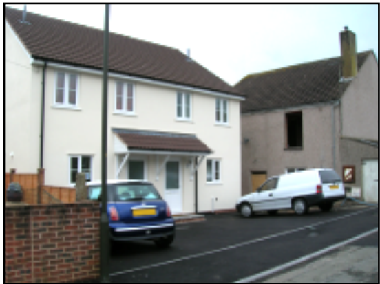
Above: the new semis at Broadwell, with what remains of the original semi on the right
