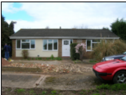
Above: completed demolition
