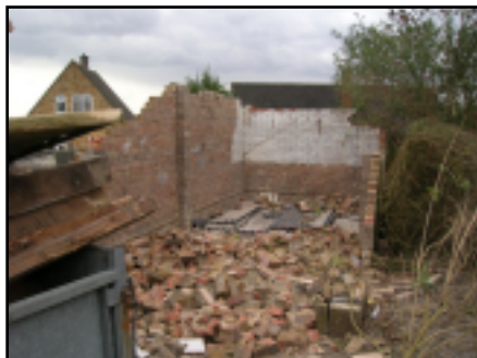
Above: garage being demolished
