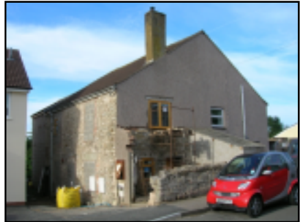
Above: the cottage with lowered wall
