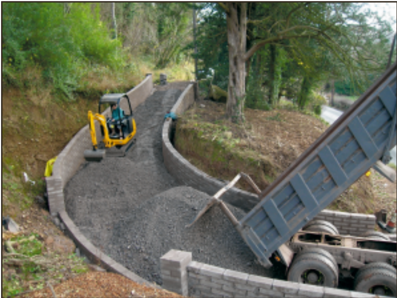
Work continues in Bishopswood
